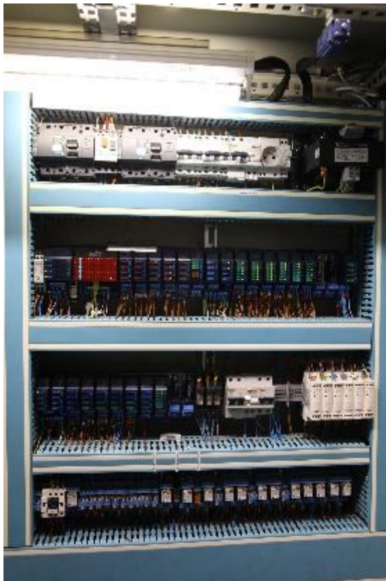
Figure 5-8: Implemented automation system on the pumping station - it works as an own EMS within the overall SCADA system. Source: EDF
