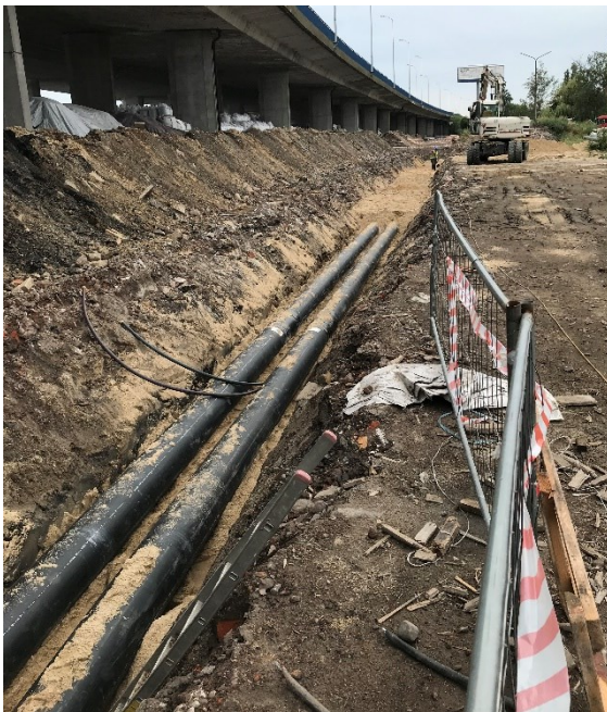
Figure 8-9: Low Temperature DH Network under Construction
