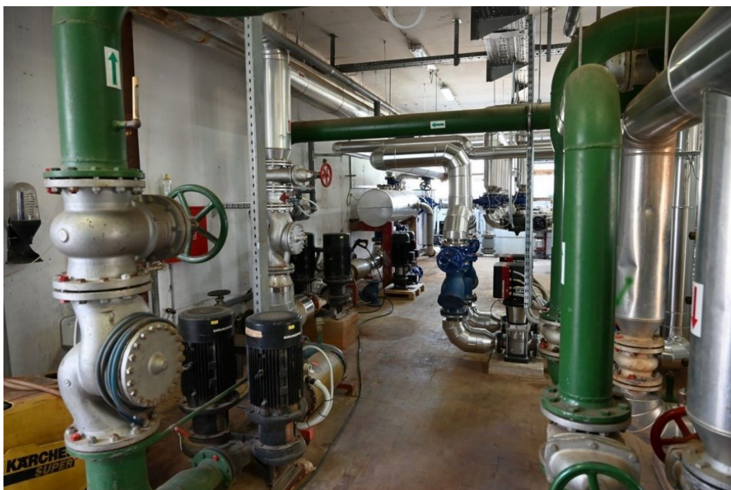
Figure 9-15: New pipelines installed at the CTS prior to flooring work
