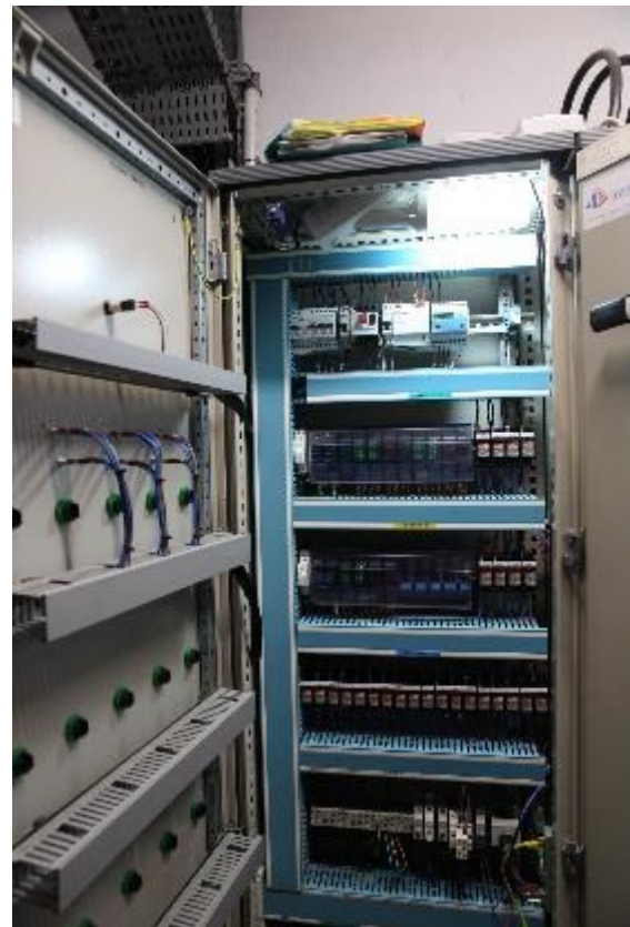
Figure 5-8: Implemented automation system on the pumping station - it works as an own EMS within the overall SCADA system. Source: EDF
