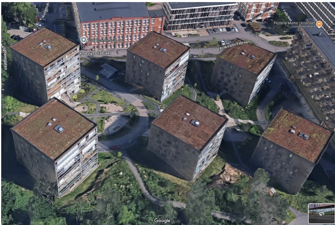
Figure 7-2: Newly connected multifamily buildings
