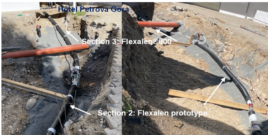
Figure 9-13: Thermaflex innovative pre-insulated plastic pipe
