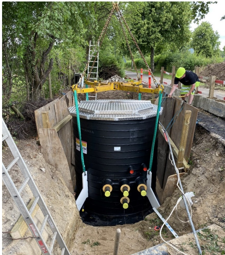
Figure 2-6: Installation of the Shunt valve - 2
