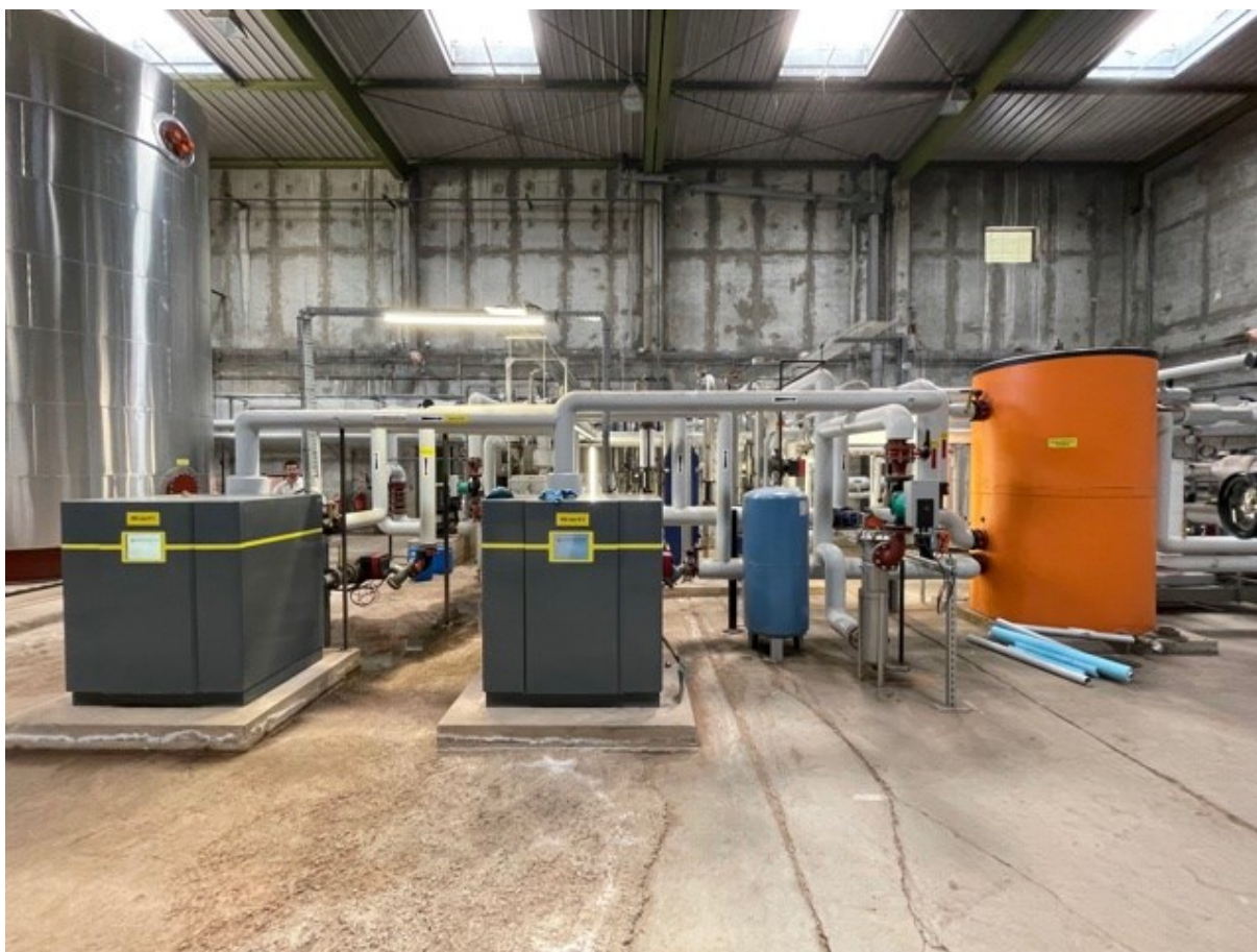
Figure 3-13: View on the main substation as operated today (Source: EDF)
