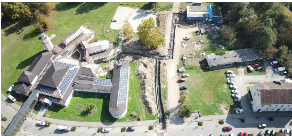
Figure 9-12: Open trench with new pipeline from CTS
