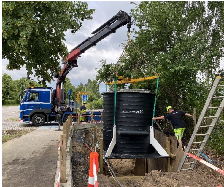
Figure 2-5: Installation of the Shunt valve - 1
