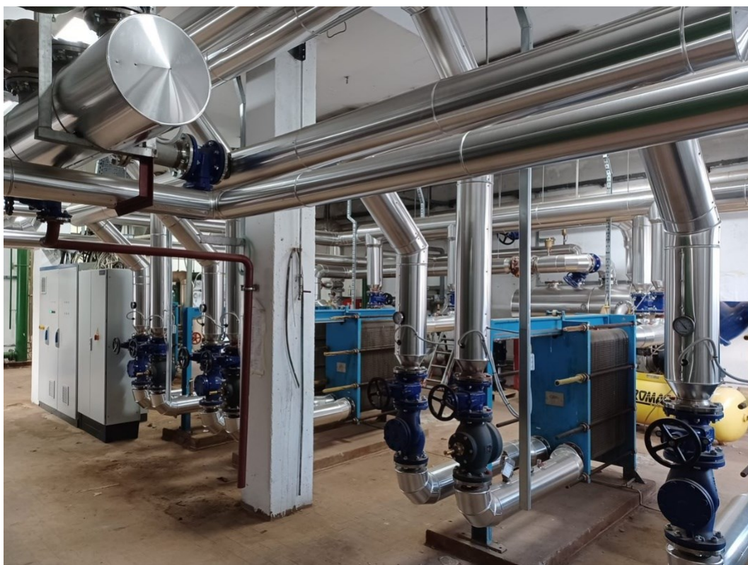
Figure 9-14: New heat exchangers installed at the CTS prior to flooring work
