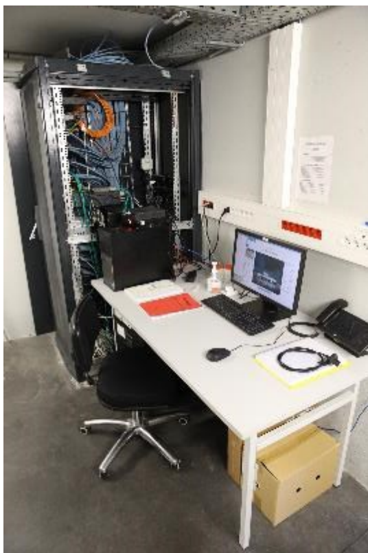
Figure 5-11: Pictures of the installed central supervision in the Armada substation and pictures of some SCADA visualizations (left: overall DHCN with its substations; right – individual substation). Source: EDF.
