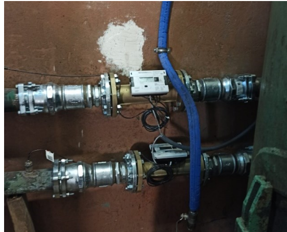
Figure 8-10: Waste heat meters at the chocolate factory, collecting data from 11.2021.
