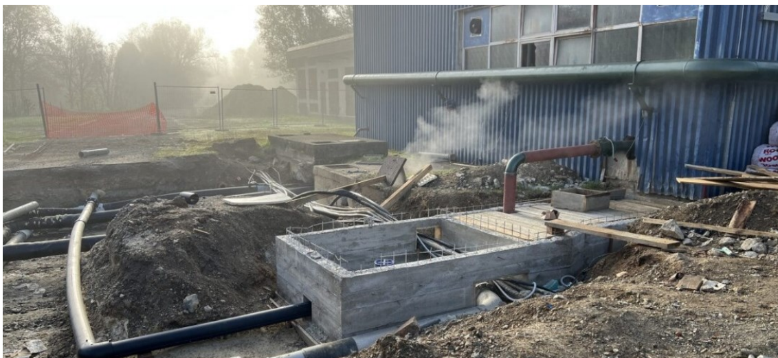
Figure 9-10: Construction works in front of CTS
