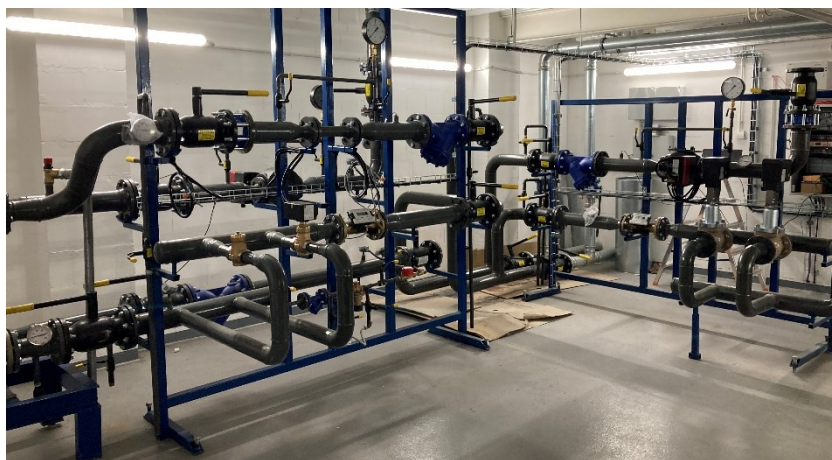
Figure 8-7: Substation under construction at the MSC
