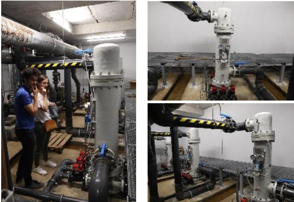
Figure 5-6: Replaced sea-water filters in the pumping station. Source: EDF.
