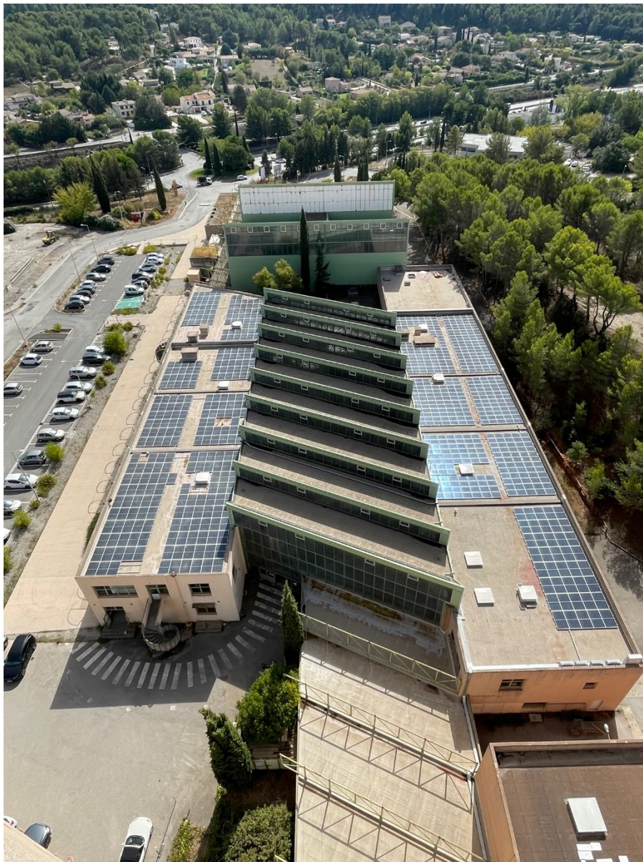
Figure 3-12: View on the House of Science and its roof-top PV field, from the top of the mine-shaft elevator tower (Source: EDF)
