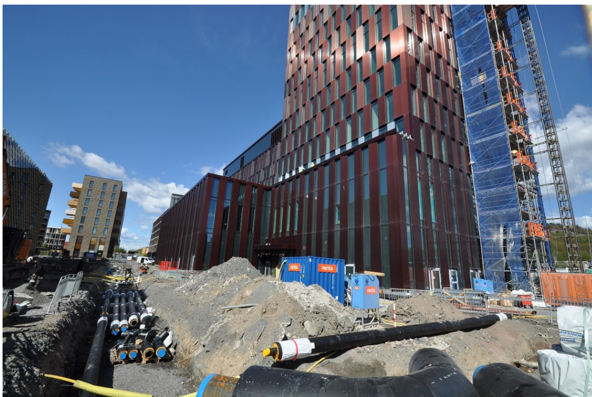
Figure 7-10: Piping Installed to Connect the Hotel to the Energy Central
